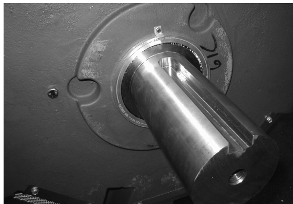
AEGIS® Shaft Grounding Ring Drive End
